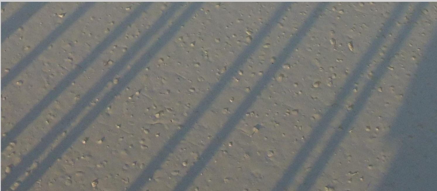
Figure 8.8. Surface finishing of SFRSCC using a cylinder shaped pipe.
