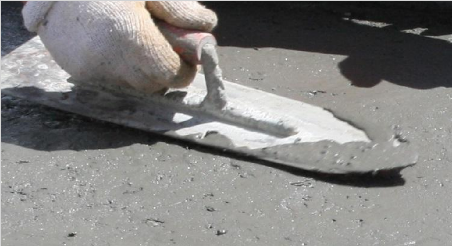
Figure 8.10. Surface finishing by manual trowelling.
