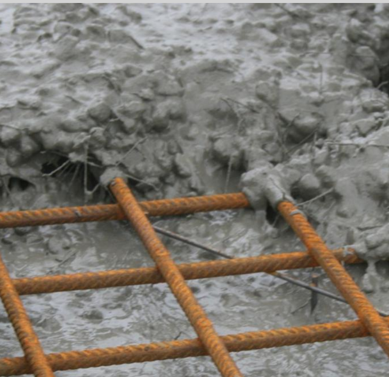
Figure 7.64. Picture of the SFRSCC close to the top reinforcement mesh.
