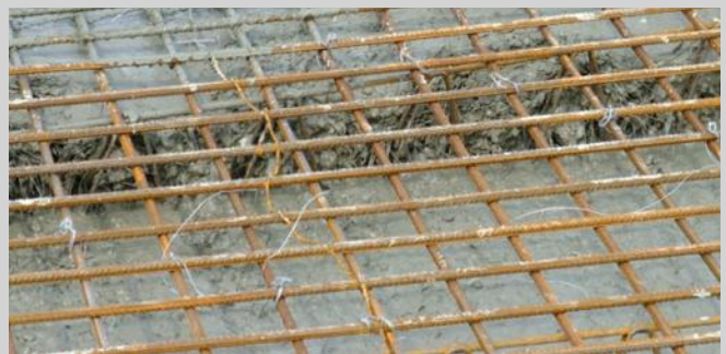
Figure 8.3: The spacer type is important to consider with respect to the risk of blocking. No blocking was observed using the spacer with a rectangular grid (top). Blocking was observed in critical areas when using a spacer type with a triangular grid (bottom).
