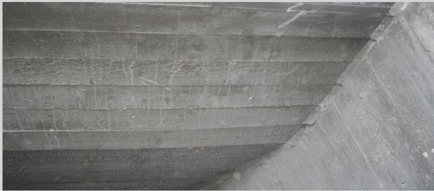
Figure 8.21: Underpass bridge. Edge beam from below.
