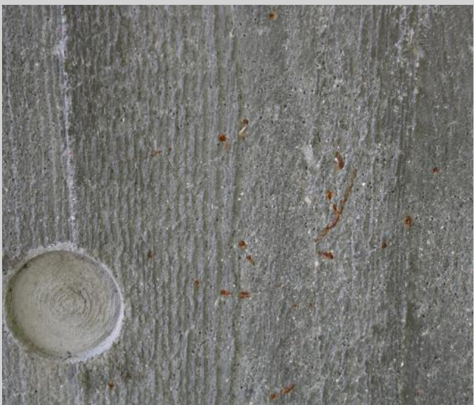
Figure 8.25: Visible fibres and rust spots on the inside walls. To the right, a fibre is sticking out.
