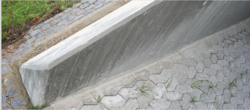
Figure 8.20: Underpass bridge. Wing wall.
