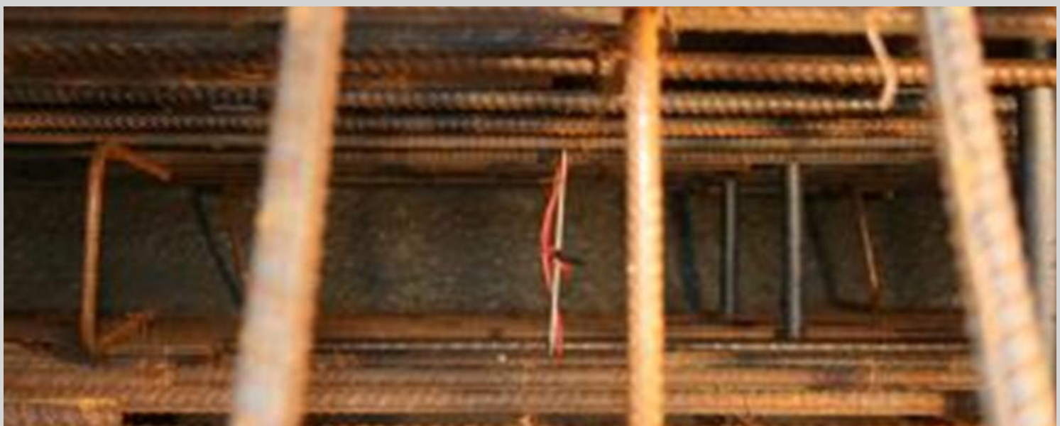
Figure 8.16: Pictures from the SFRSCC casting of the underpass bridge walls.
