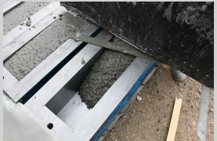
Pulling the gate. Concrete flows.
