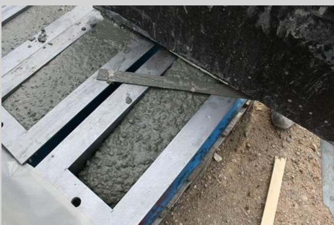
Concrete at stoppage. SFRSCC is not self-levelling.
