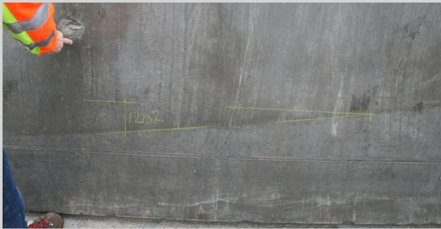
Figure 8.22: Underpass bridge. Outside surfaces.
