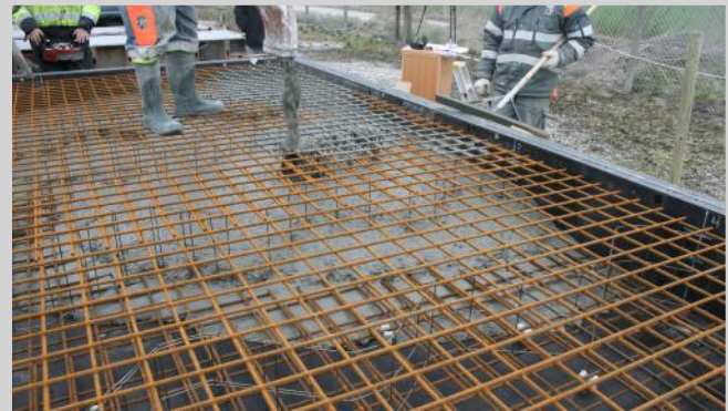
Figure 7.59: SFRSCC casting of the full-scale foundation slab (top) and trial slab (bottom).
