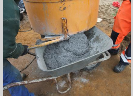
JointCast mixing on site
