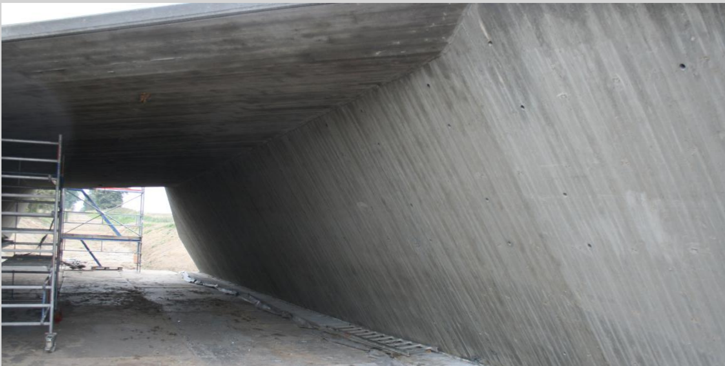
Figure 8.17: Pictures of the underpass bridge walls.
