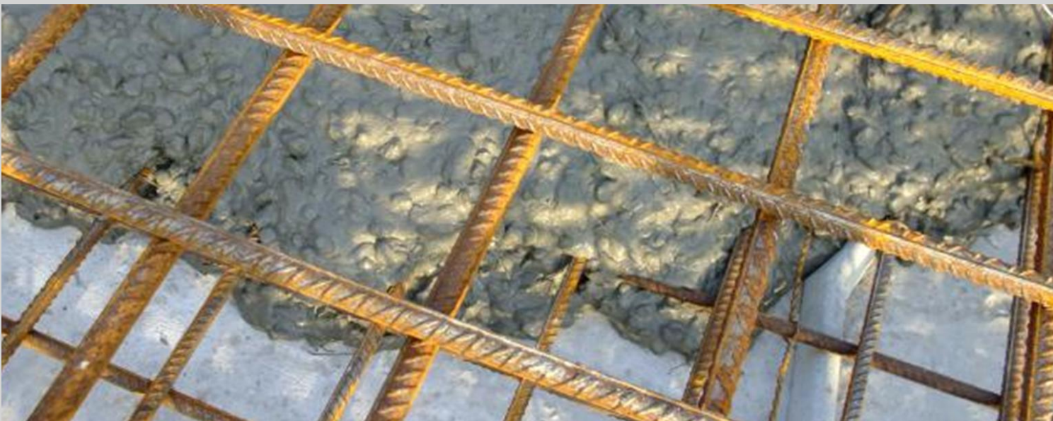
Figure 7.67. Picture from the full-scale slab casting.
