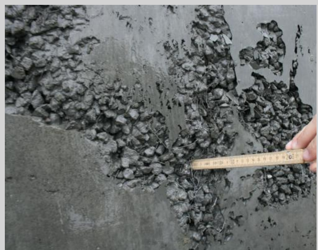
Figure 8.18: Pictures of the underpass bridge walls. Severe segregation occurred just below the cooling pipes.
