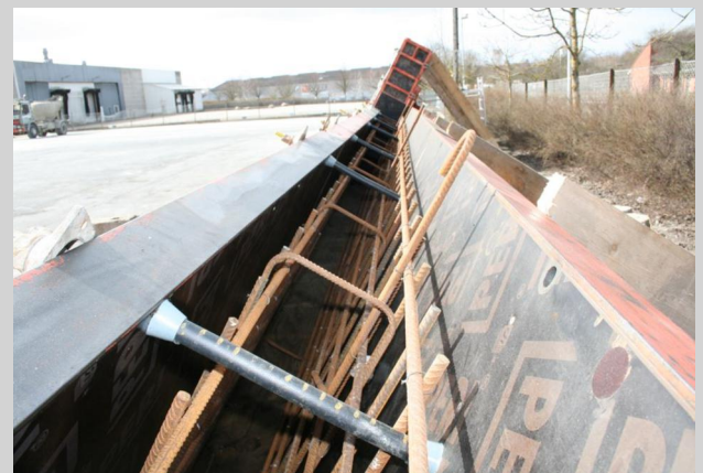
Figure 7.35: Formwork and reinforcement.
