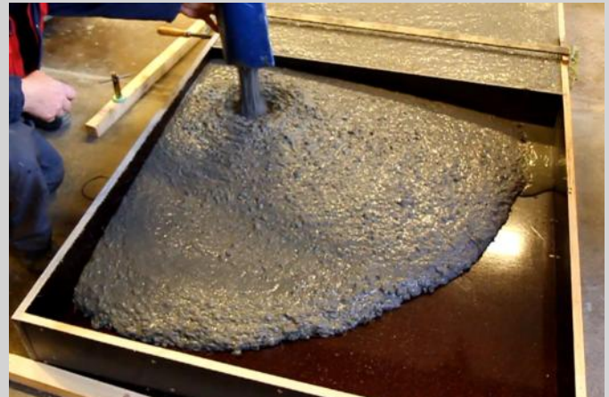
Figure 1.3: Casting of a slab with SFRSCC.
