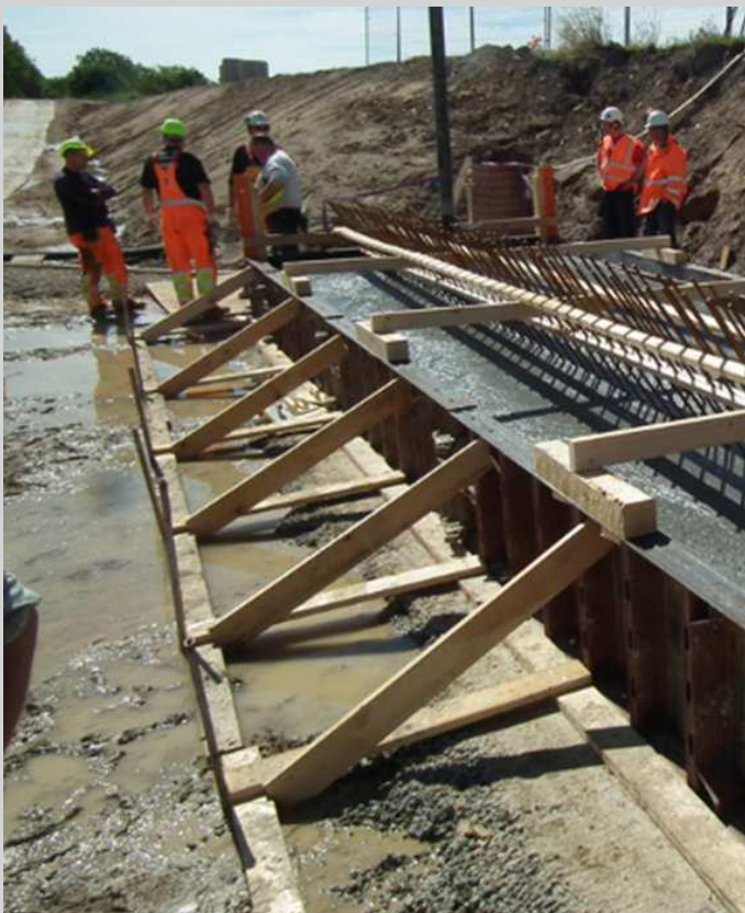
Figure 7.70. Picture from the casting of the first strip foundation.
