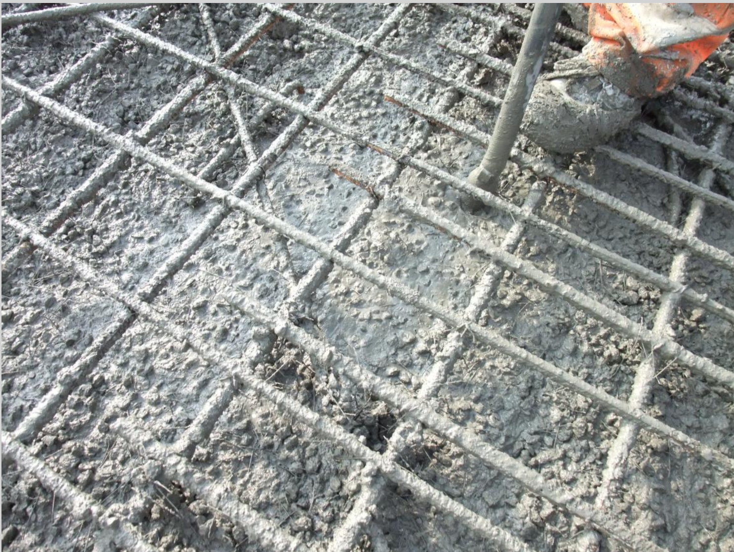
Figure 8.12. The underpass bridge deck was cast with conventional SFRC.
