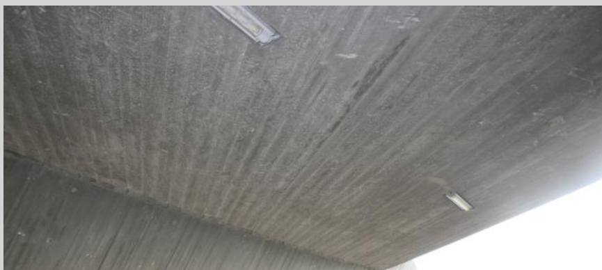
Figure 8.23: Underpass bridge. Deck from below.
