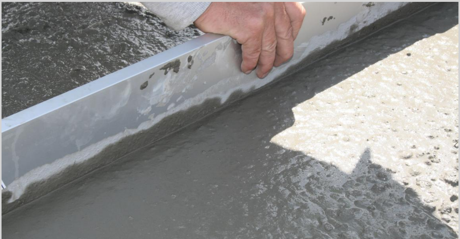
Figure 8.9. Surface finishing of SFRSCC using a screed bar.
